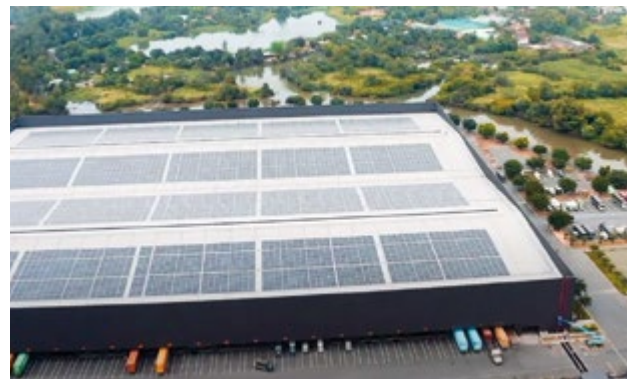
Onsite solar pannels deployed by TBS in Vietnam.
